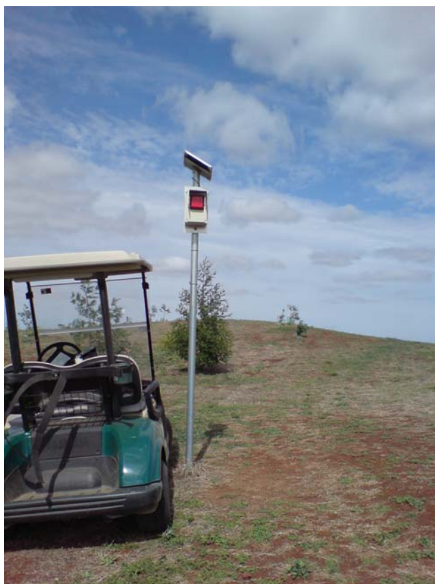
TeeSafe™ installed in a blind region on an Australian golf course.
